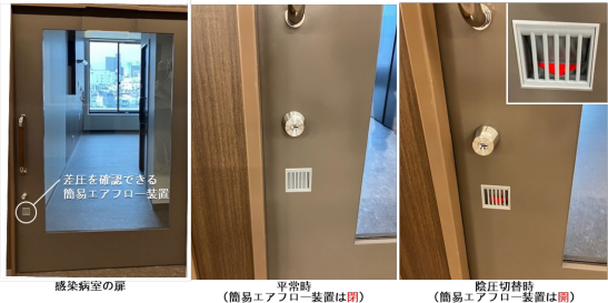
Fig.2.4.2 Status of Pressure during Negative Pressure Switching
