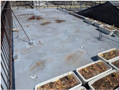
Fig.2 Rooftop on 9/11 (without planters)
