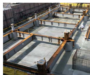
Fig.7 Foundation Construction Method without Rebar and Formwork
