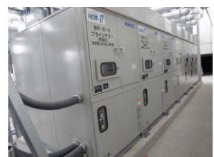
Water-cooled chiller
