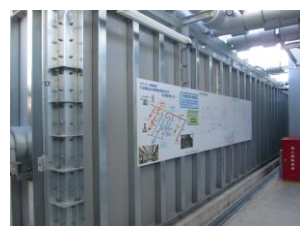
Fig.2 Ice storage tank
