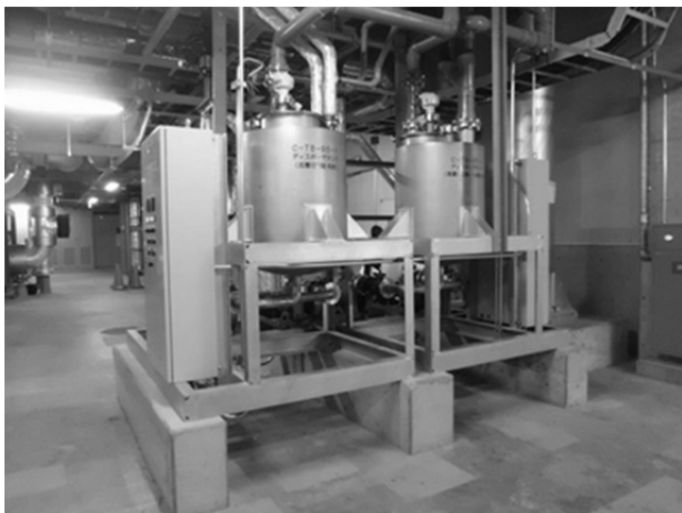
Fig.3 Disposer relay water tank
