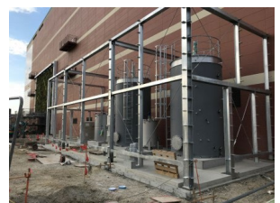
Fig.13 Fermentation tank for methane
