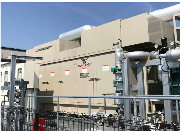
Fig.4 Gas co-generation equipment
