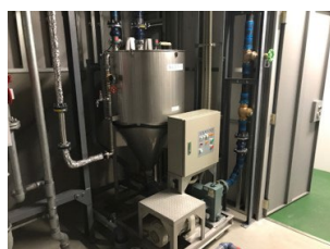
Fig.11 Relay tank for solid waste
