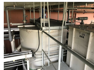
Fig.12 Pressurized flotation device to collect nutrient from waste water
