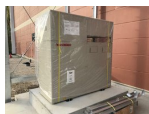
Fig.14 Co-generation used by biogas
