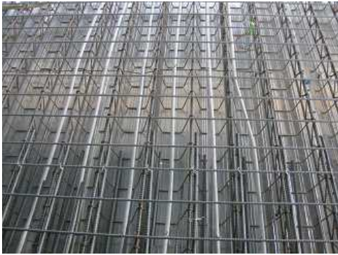
Fig-2 Buried construction situation of metal-reinforced polyethylene pipes for the Thermal Radiation Air Conditioning System
