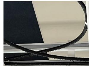
Fig. 5 Pipe Condensation
